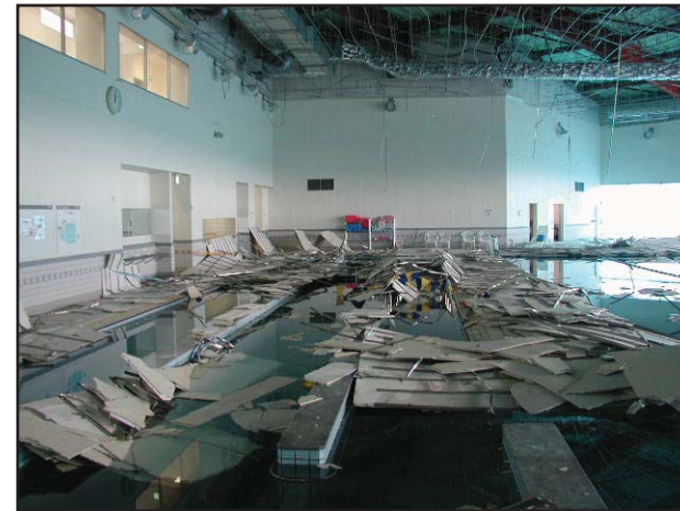
Complete collapse of the suspended ceiling over a swimming pool facility.
